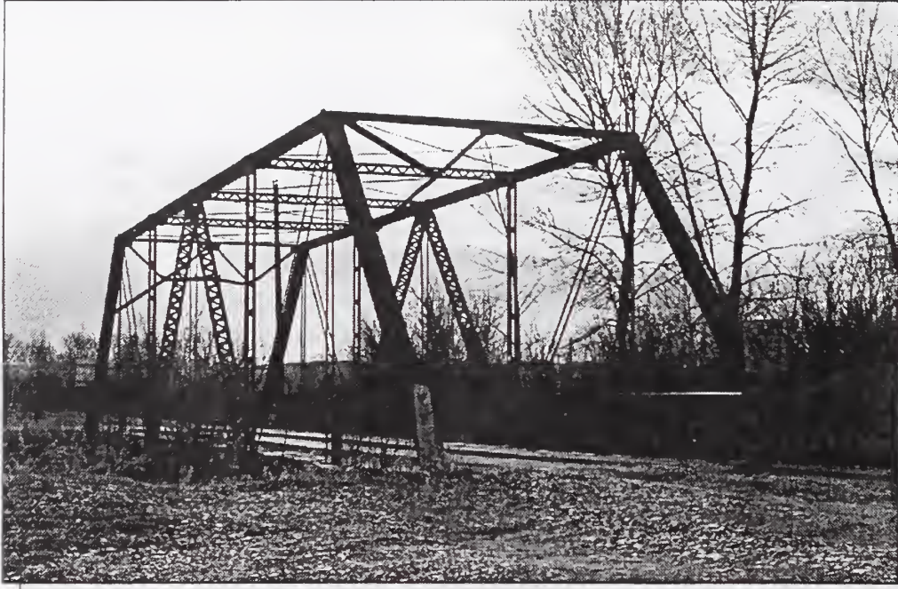
Looking Southeast from West Approach
